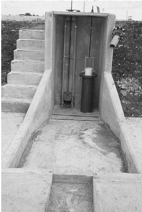
Figure 7. A concrete kettle with a catch basin in front. Note the stairway to the left, the valve that can be opened to completely drain the pond, and a moveable (up and down in this case) standpipe to control the water level when the pond is in use or being drained. The pipe on the right side of the kettle is an inflow line. The screens have been removed in this photograph.
