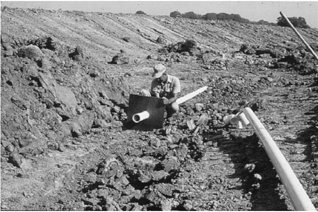
Figure 4. An antiseep collar (this one fabricated from metal) being placed around a drain line that will be installed through the levee of a pond under construction.
